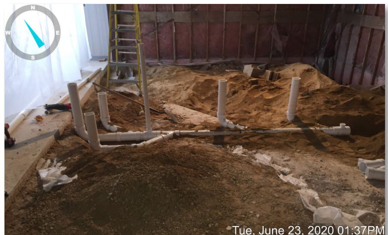
Interior plumbing for new restrooms
