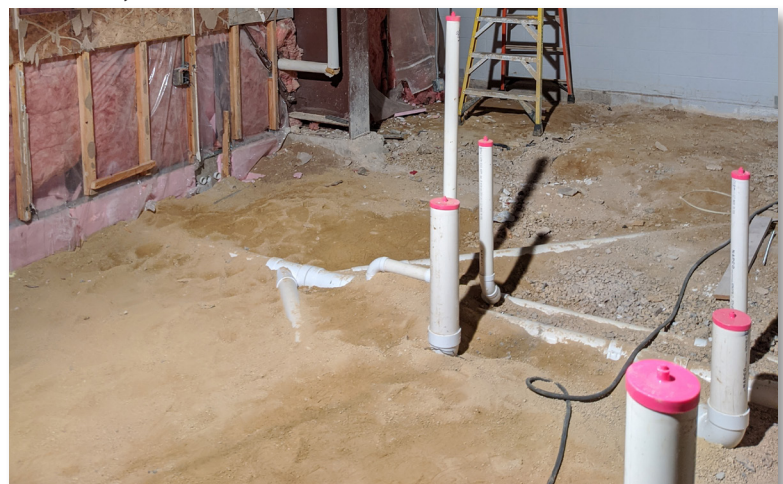
New Restroom Underground Plumbing
