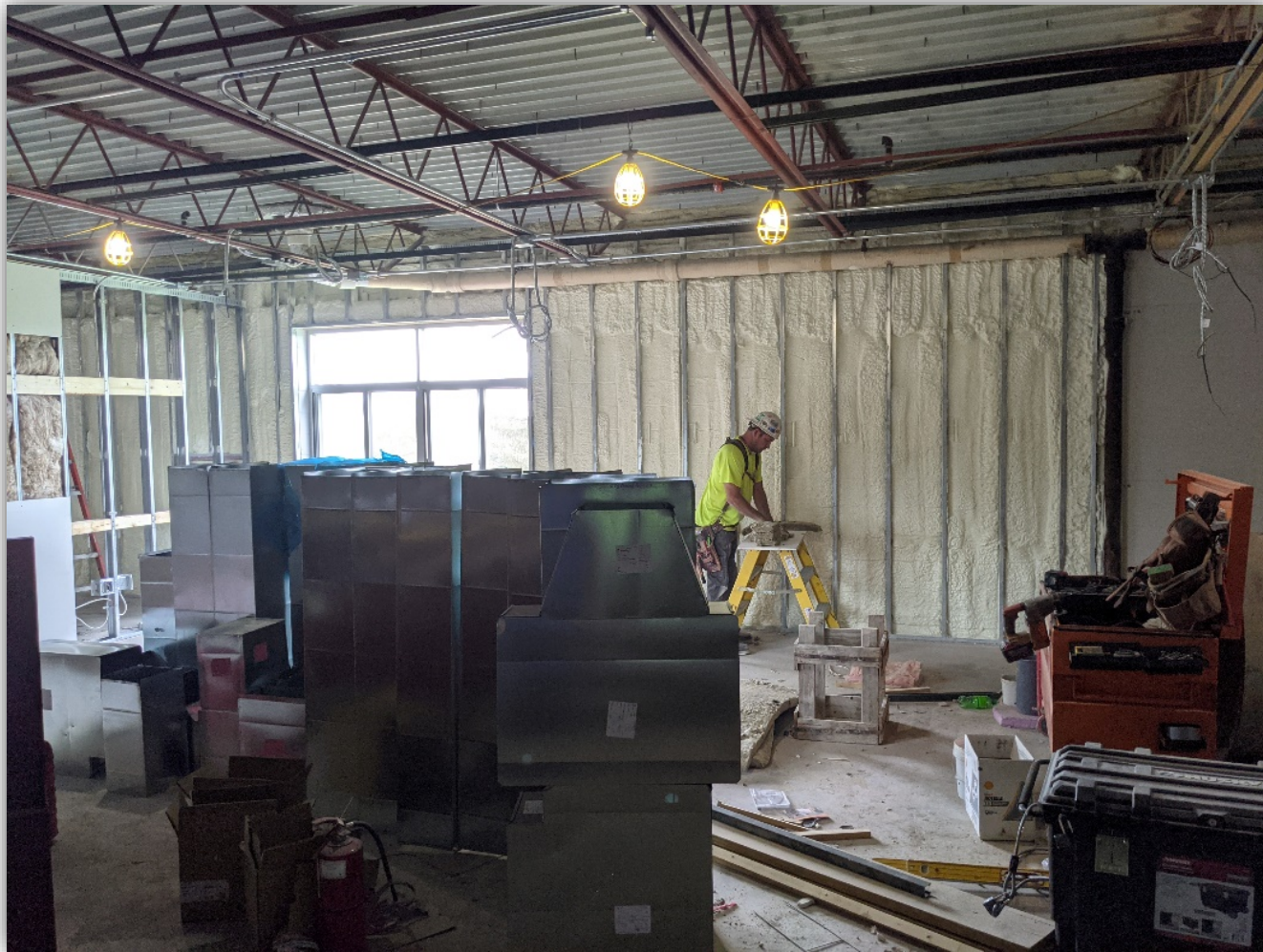
New spray foam being added on existing exterior walls
