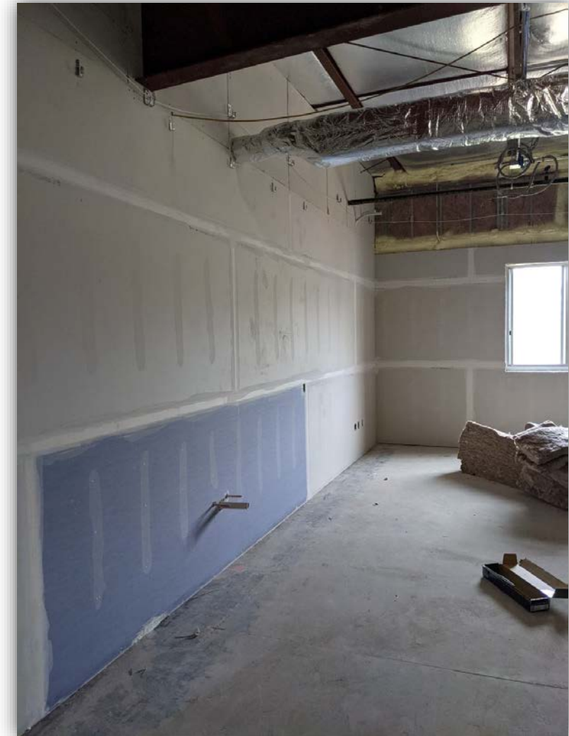
Drywall finishes being installed
