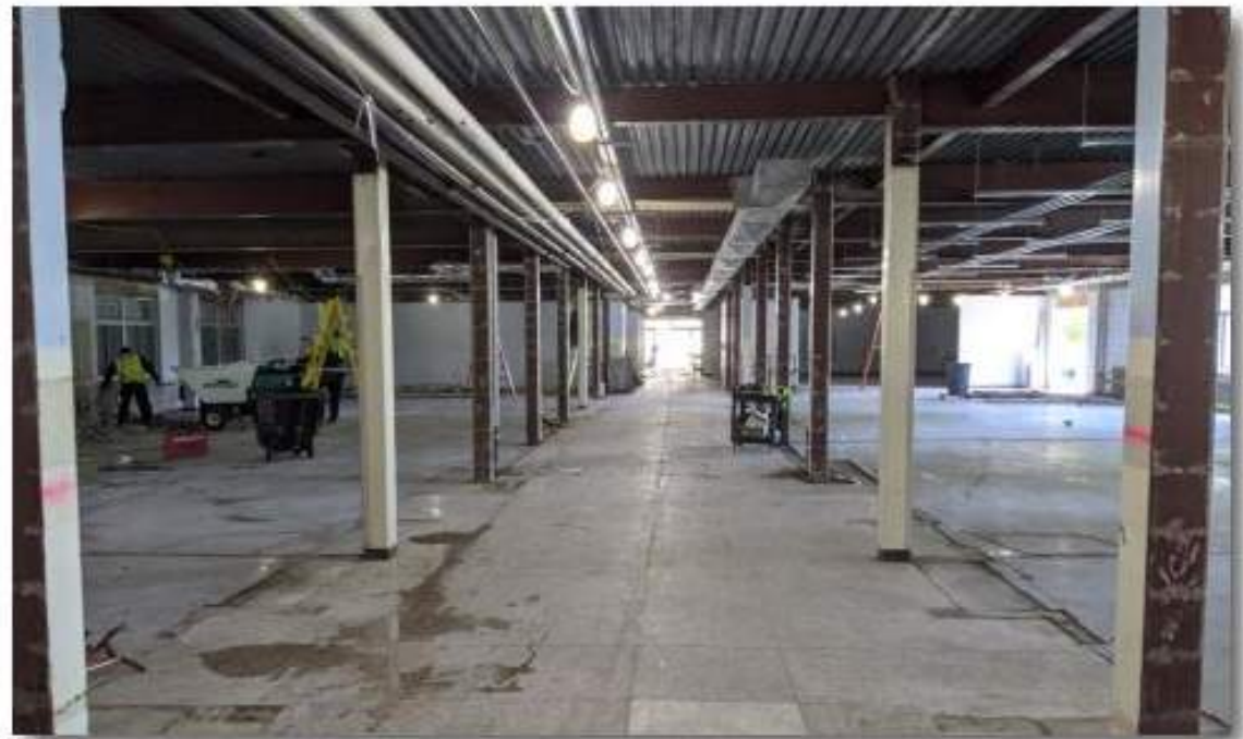
First Floor Demo Work
